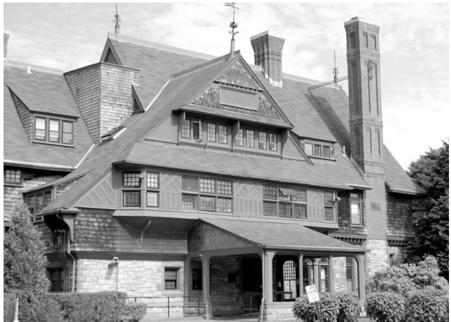
William Watts Sherman house, Newport, Rhode Island. (Henry Hobson Richardson with Stanford White, 1874-76, remodeling, McKim, Mead & White, 1880-81, c. 1900 addition by Dudley Newton). (Photo by Richard Guy Wilson)
