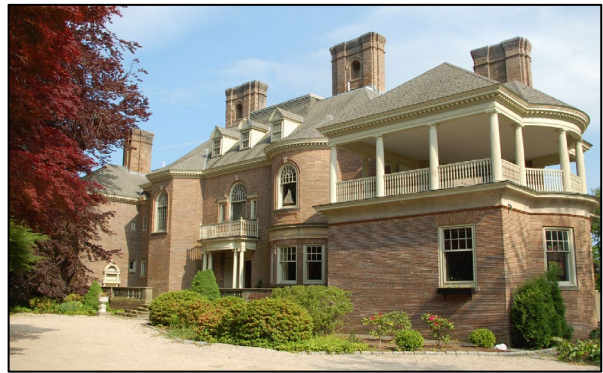
Commodore William Edgar House (McKim, Mead & White, architects), Newport, Rhode Island, 1884–86
